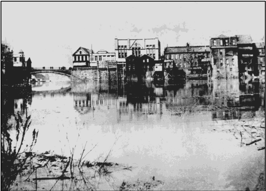
This rare c. 1870 photograph shows a flooded Krepps Bottom. To the left is the Cast Iron Bridge over Dunlap Creek, still in use today. Visible are the "stilts" which supported the rear portions of buildings along Market Street in the Neck. In 1916, Charles Snowdon converted this flood-prone bottomland into an elevated piece of real estate that he named "Snowdon Place."
