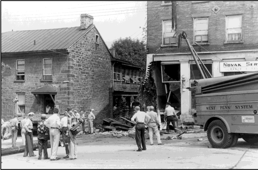
With the demolished Brown vehicle removed, the damage to the Shupe building and the Brashear House is inspected by curious onlookers.
